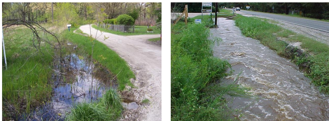
The ditch on the left, located in Kankakee County, has become clogged with growth and debris. The ditch on the right was maintained and can carry storm flows without flooding the road.
