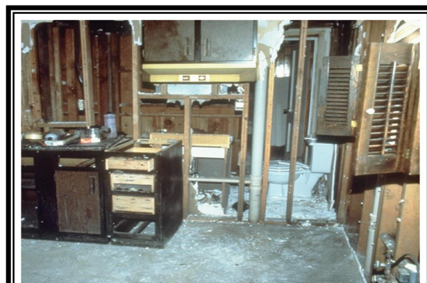
Structural flood damage includes broken walls and damage to insulation and wallboard
